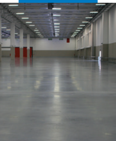
Example of industrial flooring admixed with Mapecibre NS12
